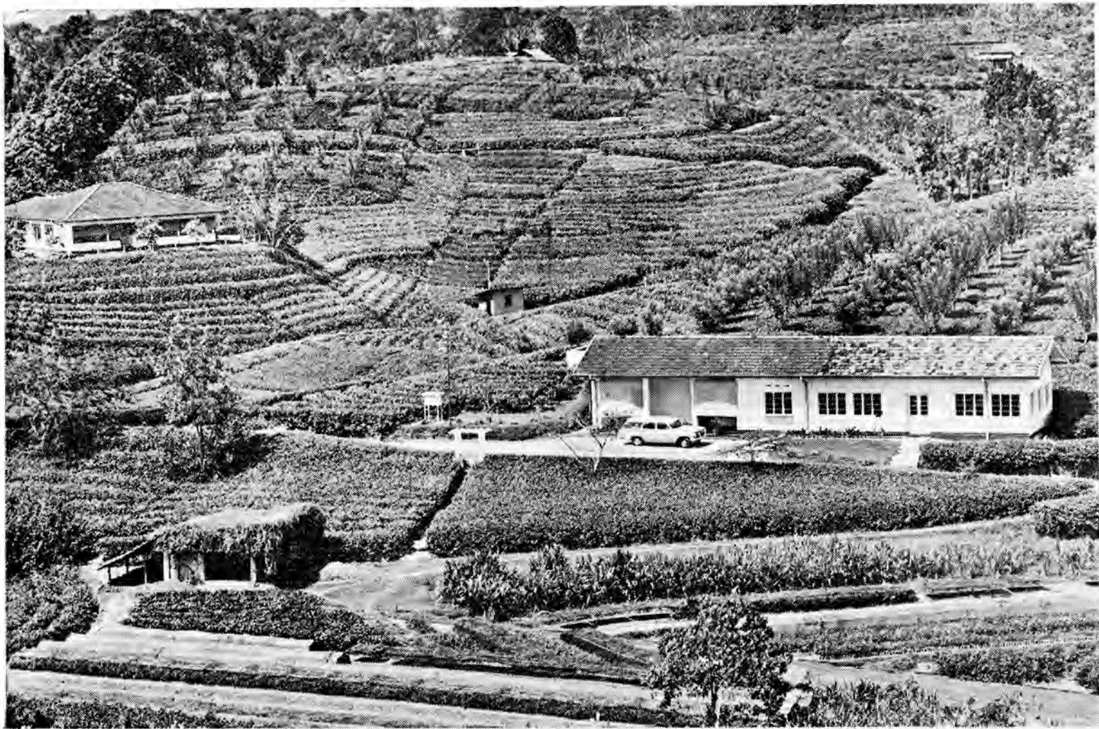
PLATE 21—The TRI Kottawa Substation, Talgampola
