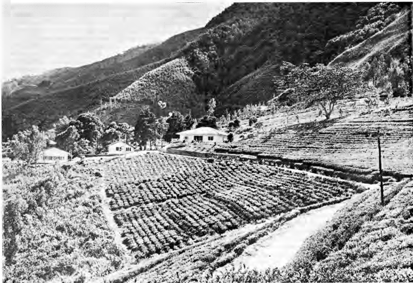
PLATE 23—The TRI Gonakelle Substation, Debedde
