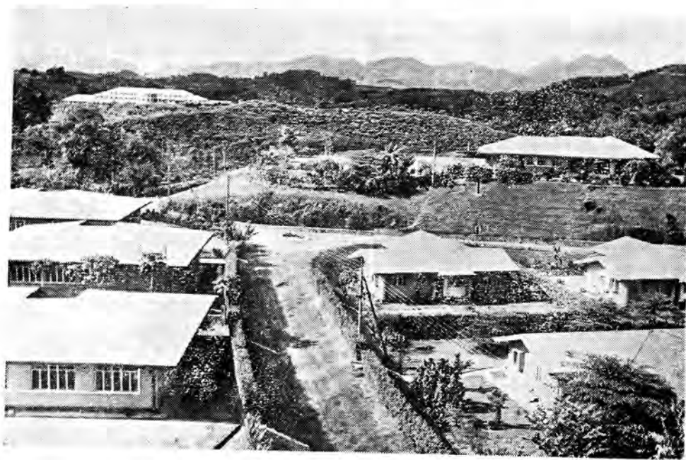
PLATE 20—Staff bungalows at the TRI Low-Country Station, Ratnapura
