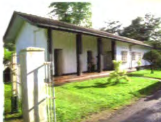
Galle (Kottawa) Advisory & Extension Centre
